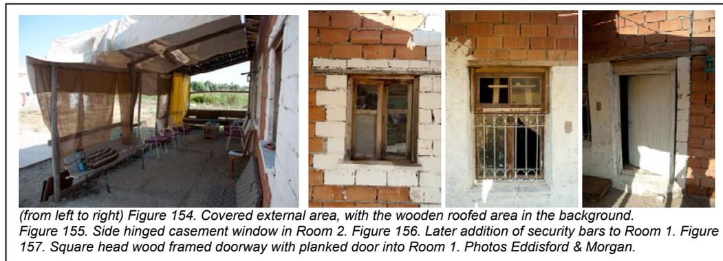
(from left to right) Figure 154. Covered external area, with the wooden roofed area in the background. Figure 155. Side hinged casement window in Room 2. Figure 156. Later addition of security bars to Room 1. Figure 157. Square head wood framed doorway with planked door into Room 1. Photos Eddisford & Morgan.
