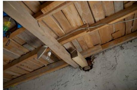
Figure 150. Timbers forming central roof support
