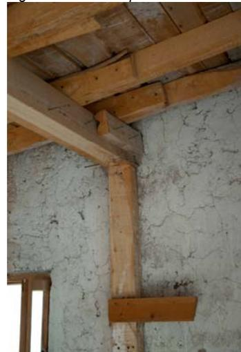
Figure 153. Vertical post for central roof support in Room 3
