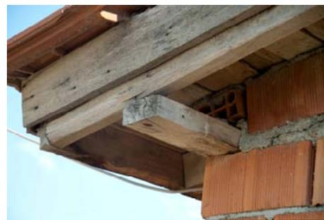
Figure 148. Wooden top beam running along the east wall.
